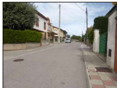
c. Montserrat (final tram 18)
