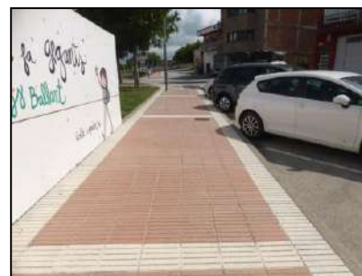
c. Major, inici vorera dreta (tram 13)
